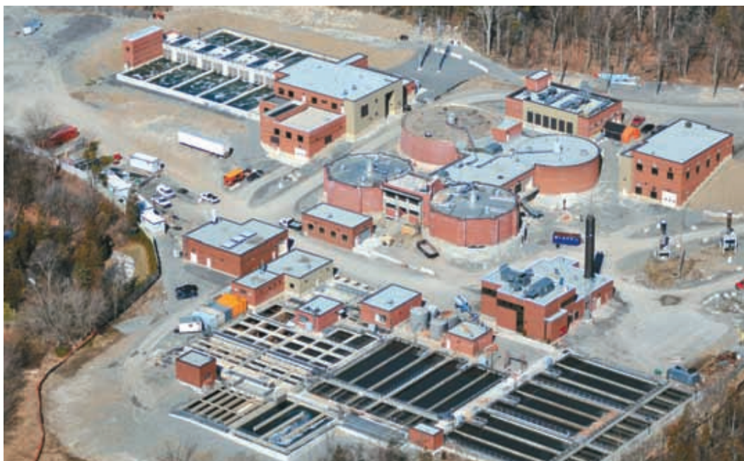
Space restrictions were a primary factor in the Ravensview Water Pollution Control Plant picking a BAF system, which upped the capacity by 30 percent.
