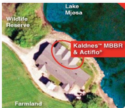
Figure 1. Skreia WWTP in Norway.
